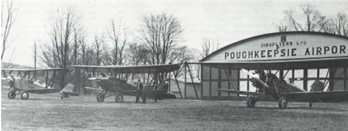
Above, John Miller's hangar at Poughkeepsie, New York with three New Standard D-25's parked in front. The center ship is Miller's D-25, NC193E, the second ship constructed by the New Standard Aircraft Company of Paterson, New Jersey. Note shorter wingspan because aircraft was assembled less the center section.
