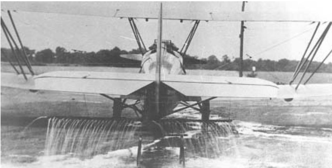
Above a very interesting spray boom installation at the aft end of fuselage under horizontal stabilizer and elevators. Normal installation favored area below the lower wing. Photo from Steve and Kathleen Maciag.
