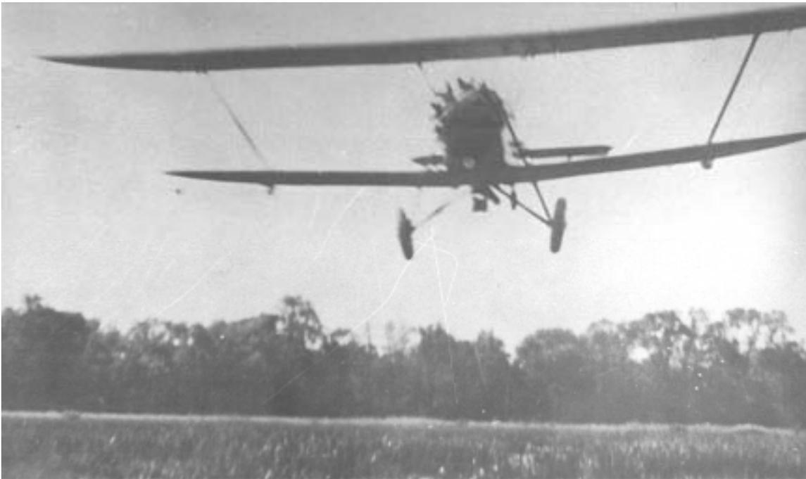
Above, a New Standard D-25 powered with a Wright J-5 engine at work. Caption on back of each photo states, “Spraying mosquitoes in Morris, New Jersey, 1930’s.” Photos obtained from Steve and Kathleen Maciag.
