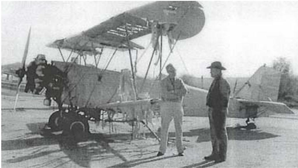
Carl Small visiting with Dick Comfort next to New Standard D-25 at Fram Field near Phoenix, Arizona. Note condition of structure and fabric covering also conversion to BT-13 hydraulic wheels and brakes. This aircraft also went to Old Rhinebeck Aerodrome in New York. Max Shear sold 5-ships in deteriorated condition to Cole Palen at Old Rhinebeck. Two of those aircraft have been restored and are now flying. Photo from Carl Small
