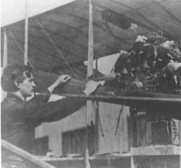
engine of his design using five-Harley Davidson cylinders arranged in a semi-radial fan configuration. Tractor design indicates propeller pulls the ship through the air, as opposed to a pusher design that pulls the ship through the air. Day flew the craft unsuccessfully near Playa Del Rey, southwest of Los Angeles. He repaired the craft and flew successfully at Dominguez Ranch, south of Los Angeles.
